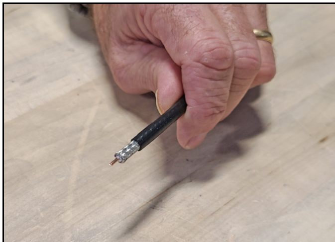
Figure 50: Cable Stripped, Exposing Dielectric
