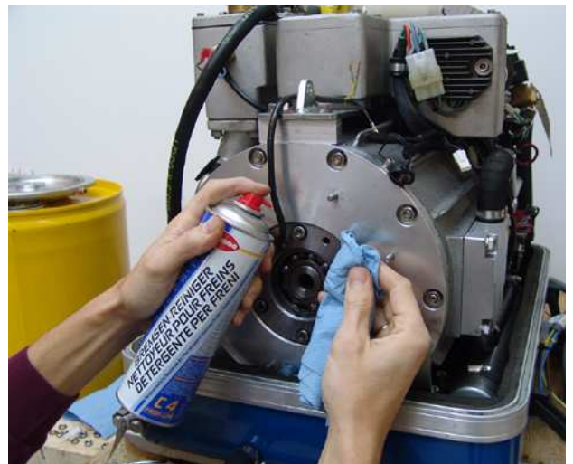
Fig. 6.10.2-4: Marking the bearing position
